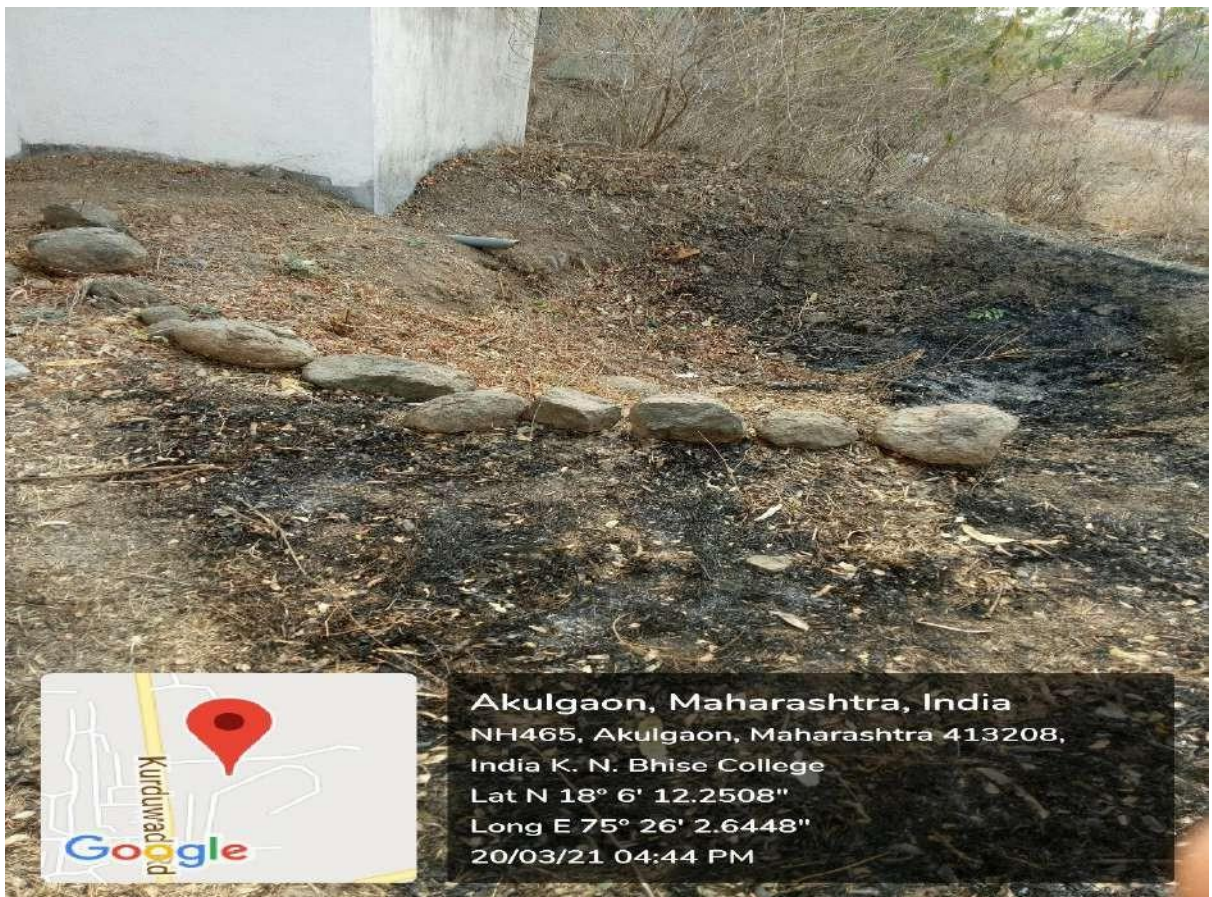
Hazardous Chemical Wastage Outlet
