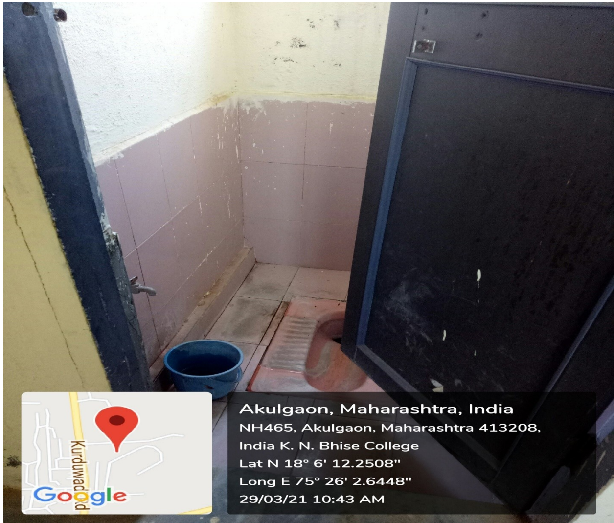
Toilet Facility in Ladies Common Room
