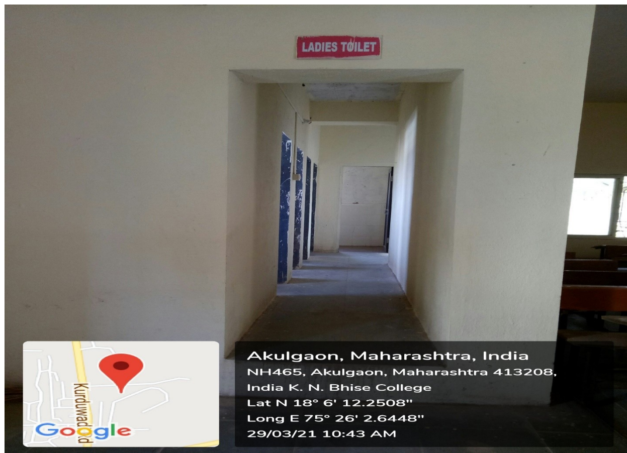
Toilet Facility in Ladies Common Room
